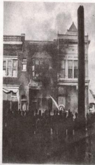
By 1 p.m., smoke billowed out of the building so thickly that no one could determine exactly where the fire was located.
