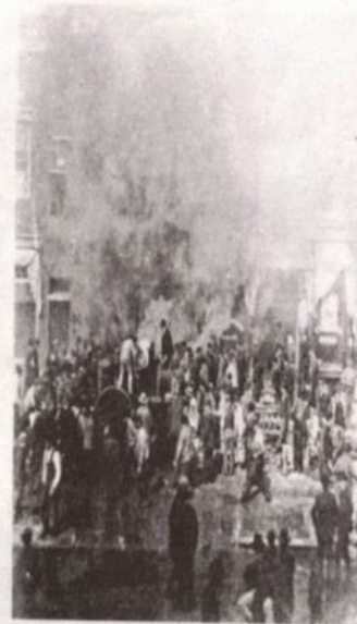
Howell's only piece of fire equipment, the Champion Fire Extinguisher, and hundreds of men carrying buckets of water went to work attempting to put out the fire. Meanwhile, merchandise from H. C. Brigg's Jewelry Store and F. K. Johnson's Drug Store, the two stores on either side of the grocery, was moved onto the courthouse lawn.
